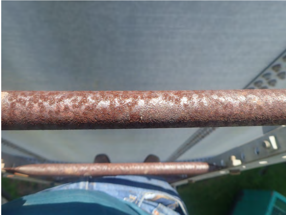
Photo 11: Exterior ladder rungs with corrosion
