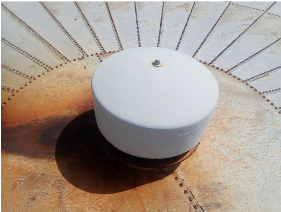
Photo 14: Vent with corrosion and staining
