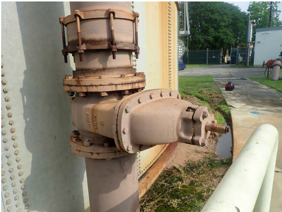
Photo 10: Fill line with corrosion
