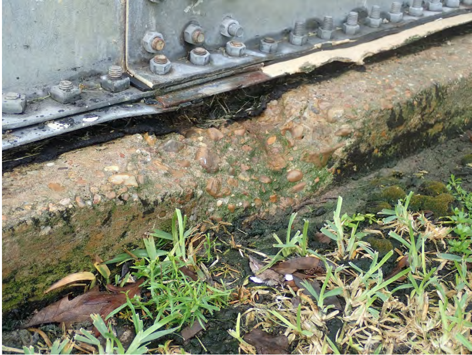
Photo 1: Foundation with spalling
