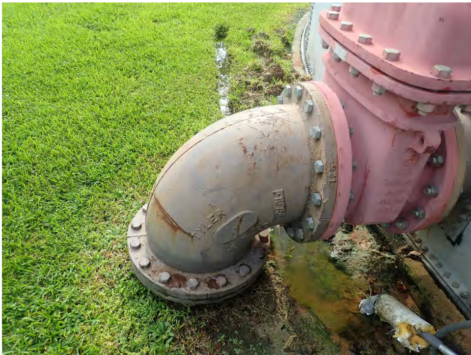
Photo 6: Suction line with corrosion
