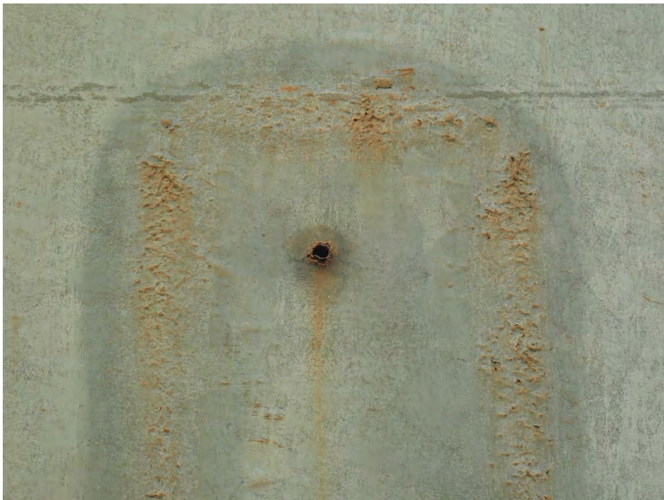
Photo 4: Exterior wall panel with corrosion
