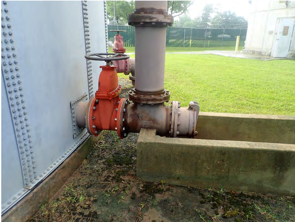
Photo 7: Overflow/drain line with corrosion
