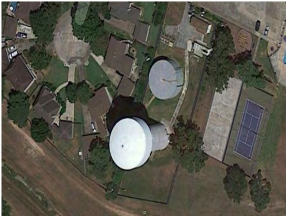
Water plant site overall
