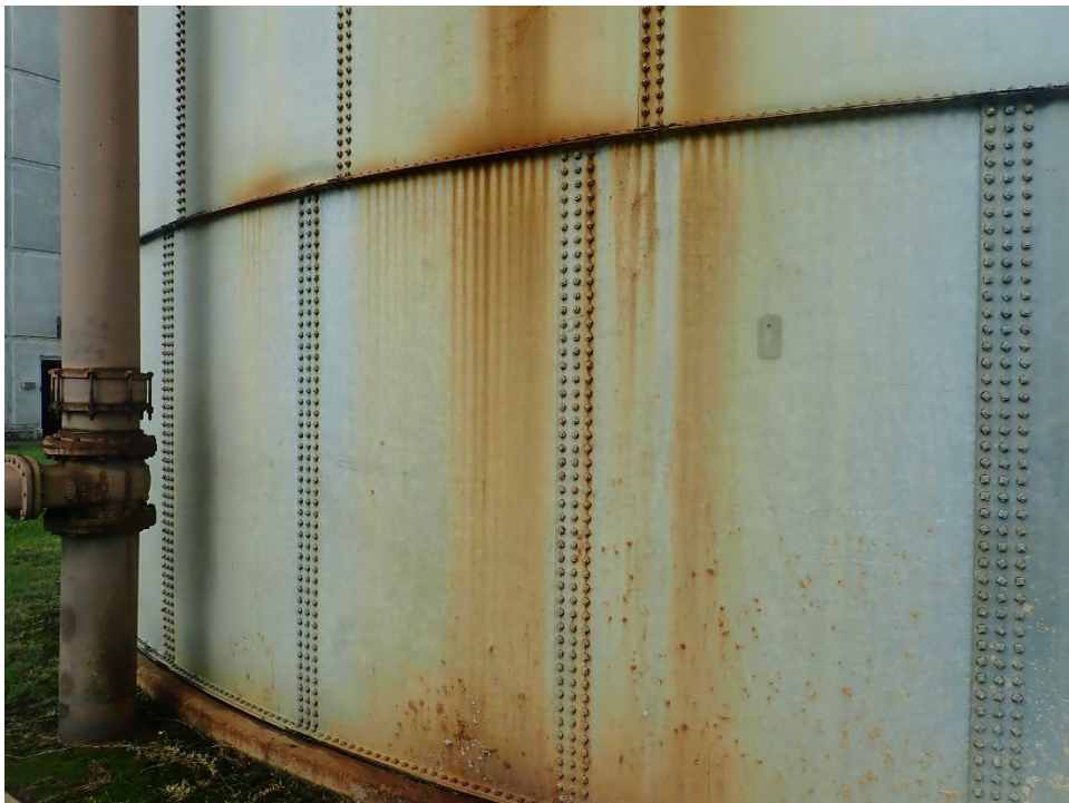
Photo 2: Exterior wall panels with staining and corrosion
