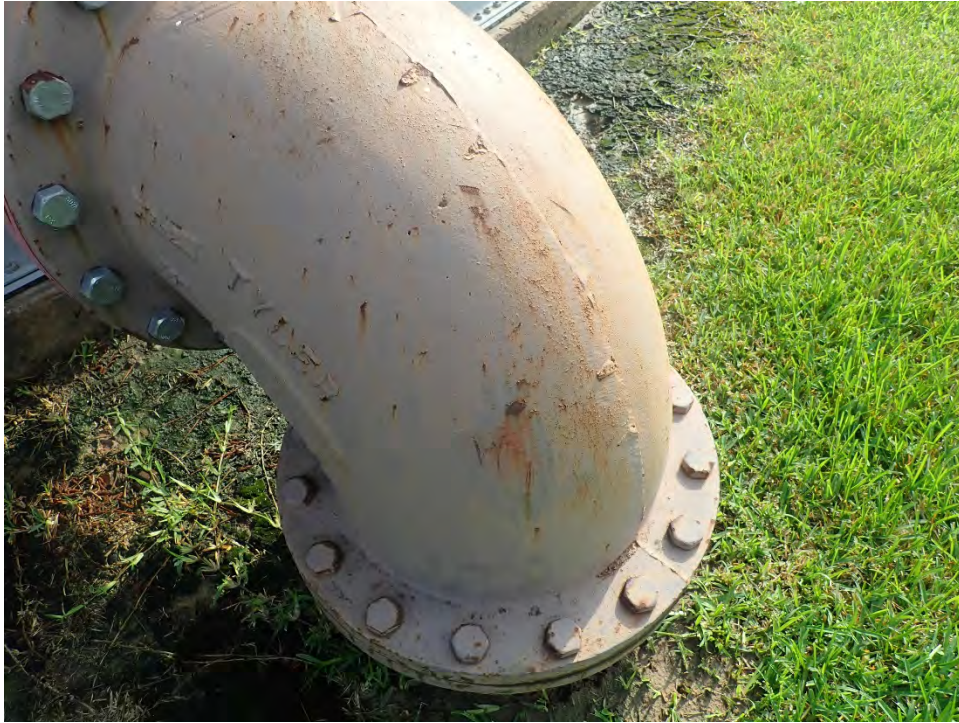
Photo 9: Suction line with corrosion
