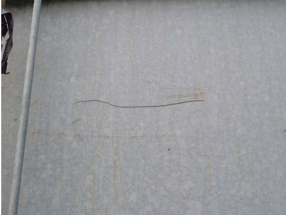
Photo 3: Exterior wall panel with corrosion
