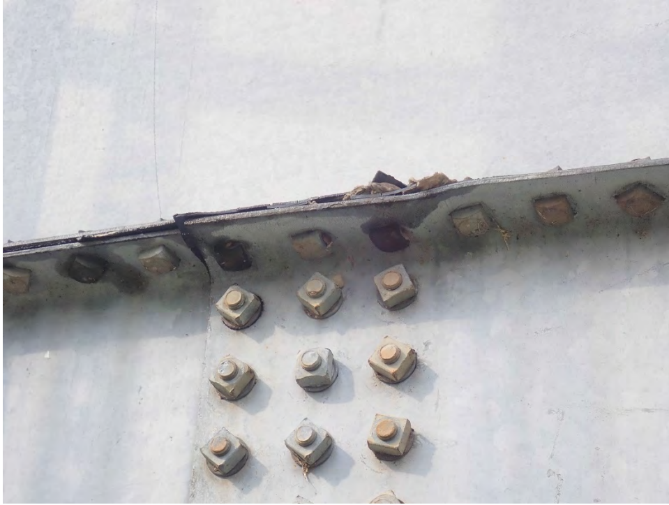
Photo 5: Bolt strips with corrosion
