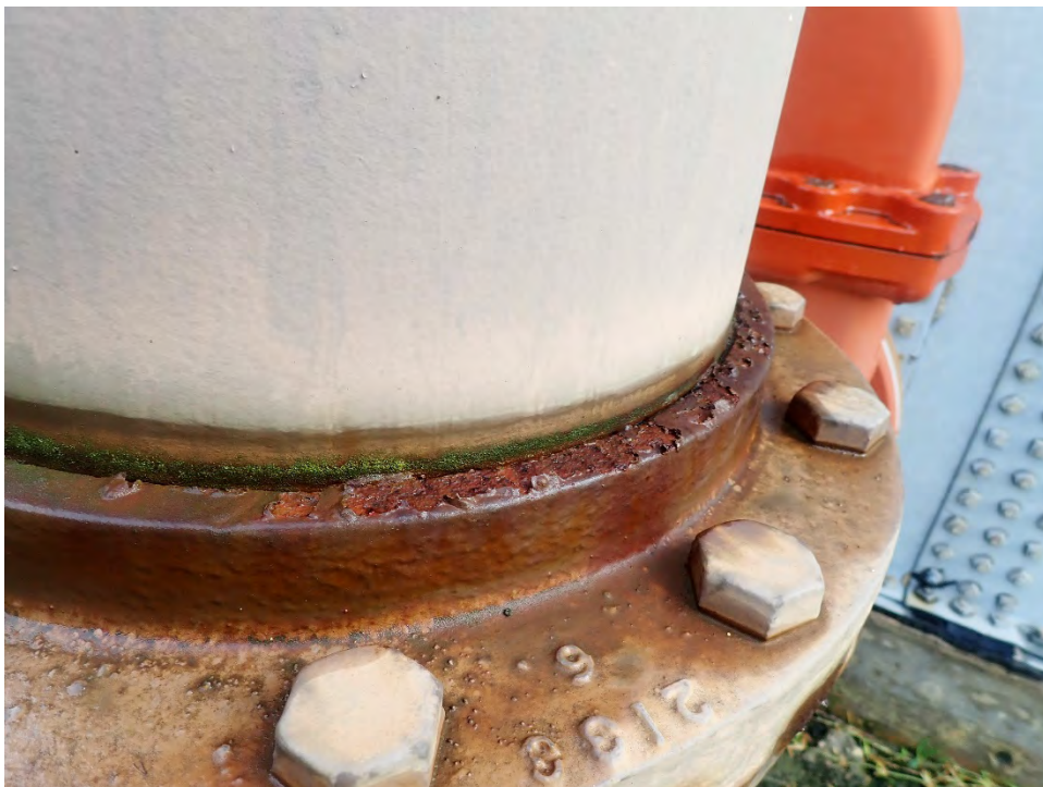
Photo 8: Drain line with corrosion
