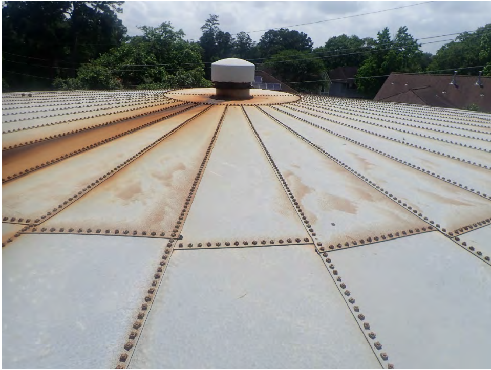
Photo 13: Roof panels with corrosion
