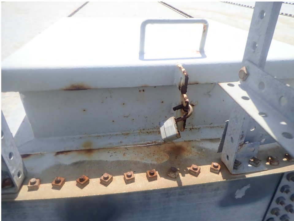
Photo 12: Roof at hatch with corrosion
